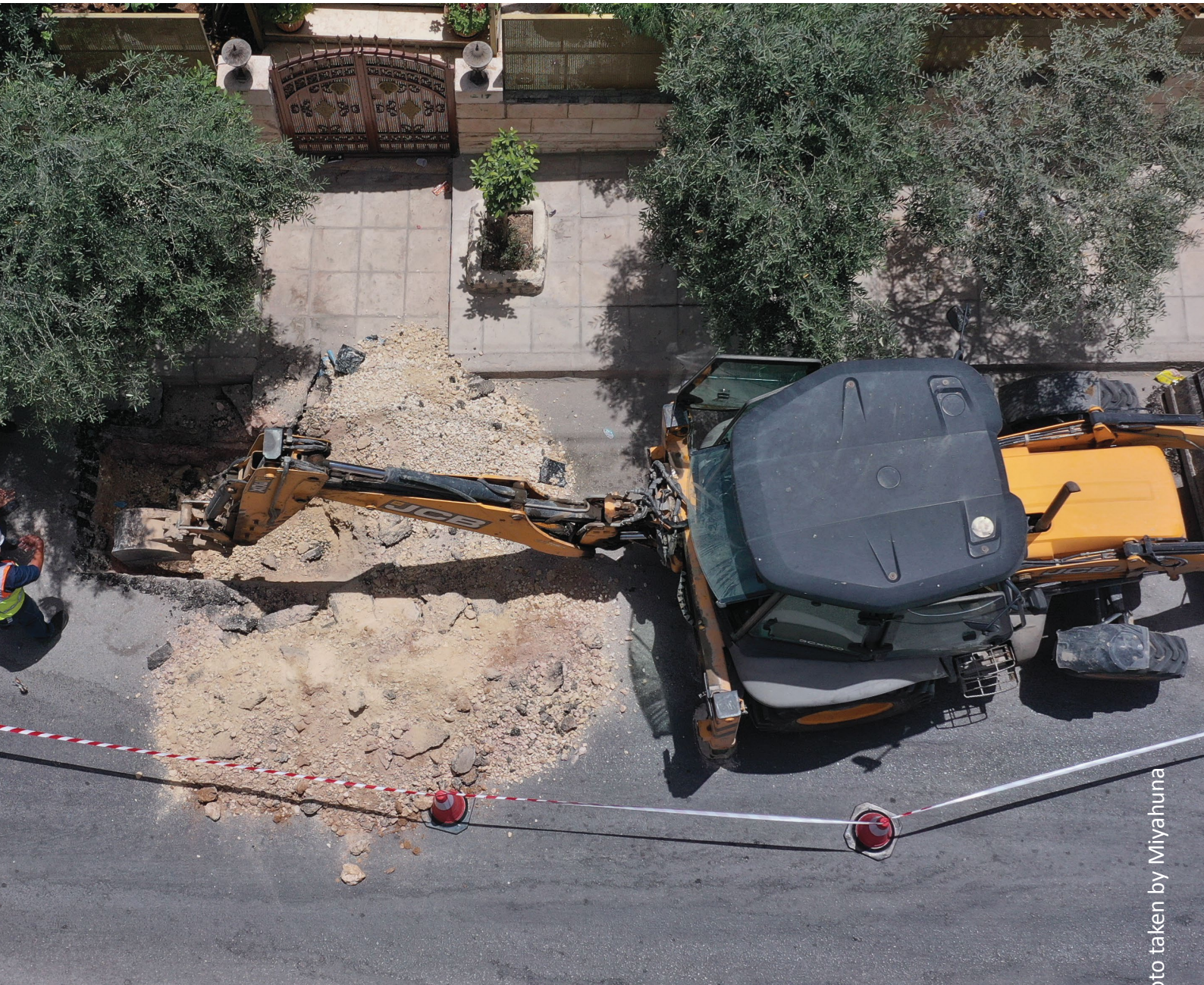
An aerial view of repairing a water pipe in Amman Governorate
